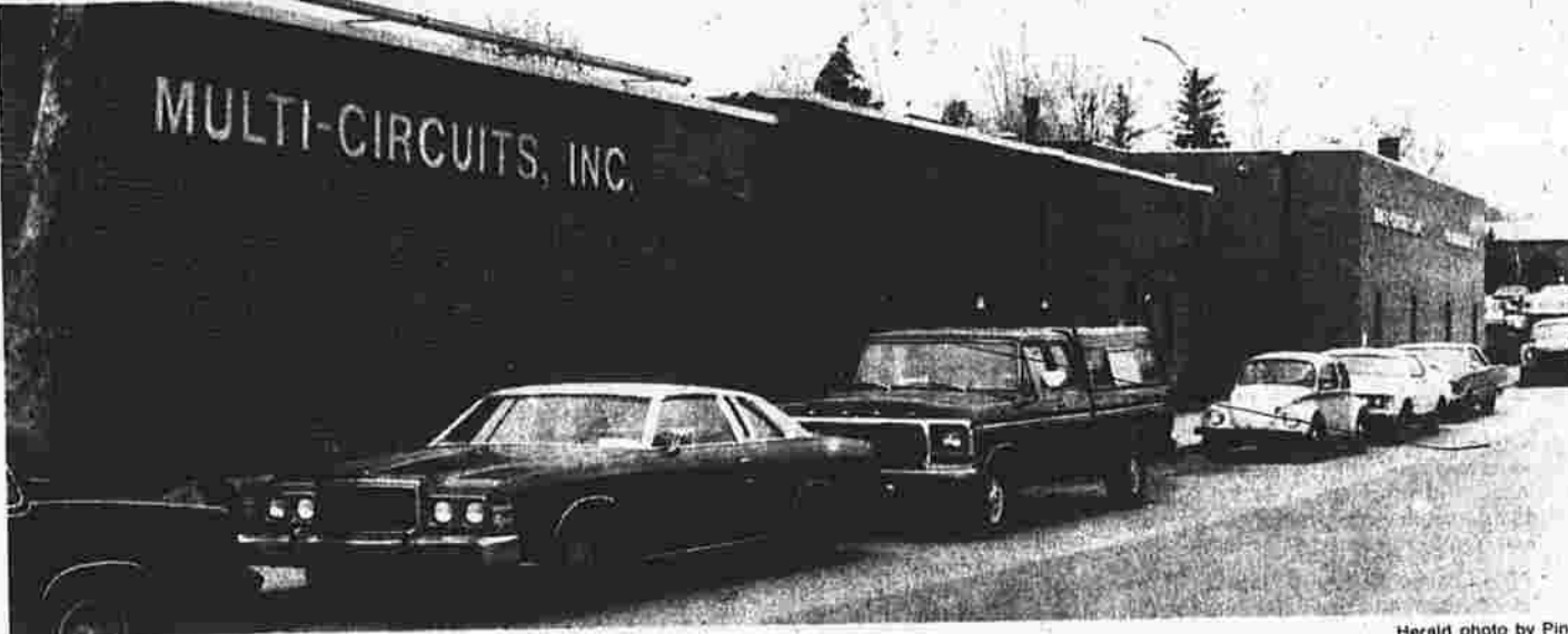
Employees' autos line the side today of the Multi-Circuits building on Harrison Street.
